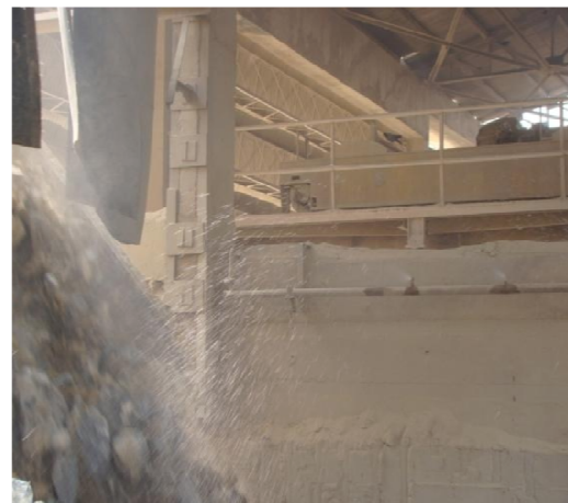
Photographs of Water sprinkling system at limestone handling
